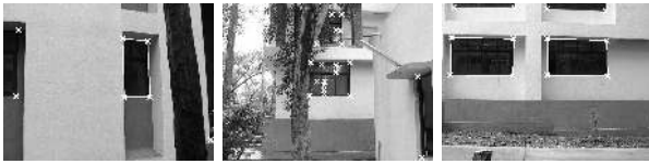
Fig. 13. Experiment 7 (I.I.T. Bombay buildings): Catastrophic failure - the effect of an occlusion (left), and reflection on the window panes and tree (centre) (details in text.)
